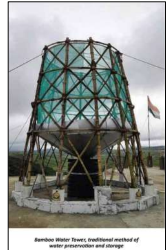
Bamboo Water Tower, traditional method of water preservation and storage
